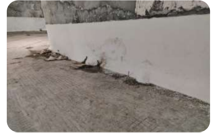
Coating on walls for waterproofing
