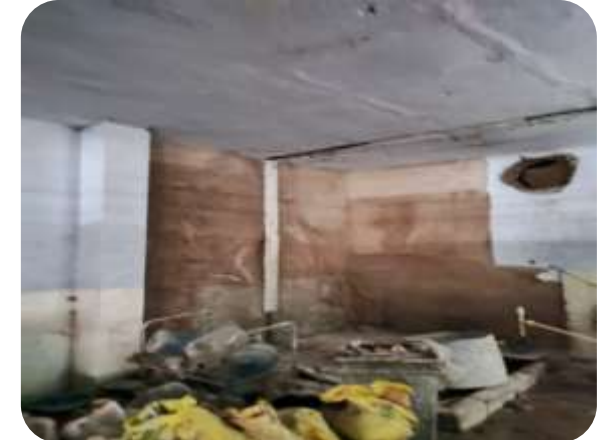
Expansion joint Area.
