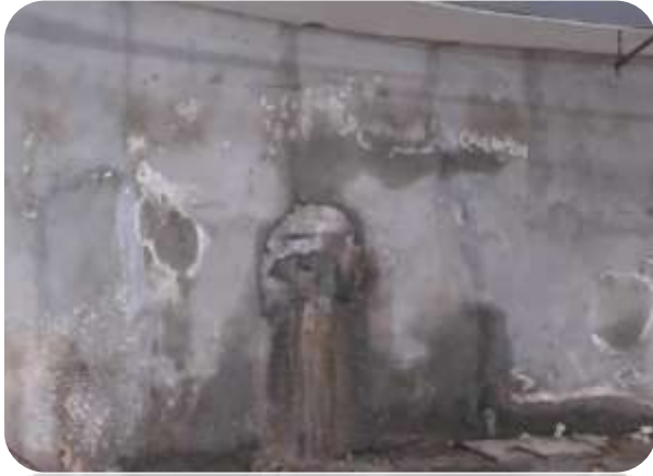
Drying of walls after grouting.
