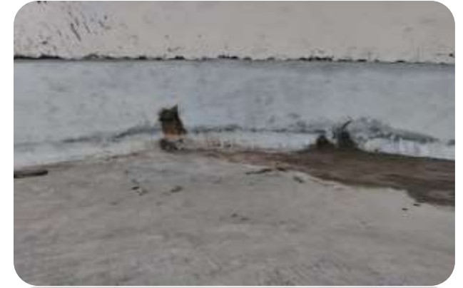
Joints of RCC
